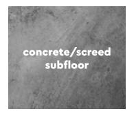
**Let new concrete dry sufficiently.** The moisture content of the subfloor must be less than 75% RH at min. 20°C. Max 2% CM for cement and 0.5% for anhydrite.
